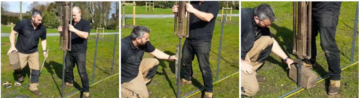
Drive the post in a couple of inches then use a spirit level to upright before driving in the rest of the way. Use a wooden block and align with the bottom hole in the fence post to set a height. This should be an inch or so higher than the finished height.
